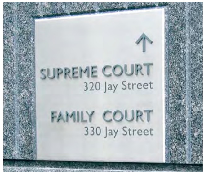
Cutout stainless steel letters on stainless steel plaque
